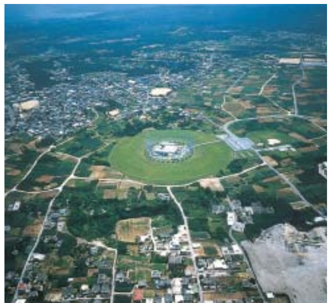
The antenna facilities at Sobe Communication Site (dubbed the "Elephant Cage"), which will be relocated to Camp Hansen.
