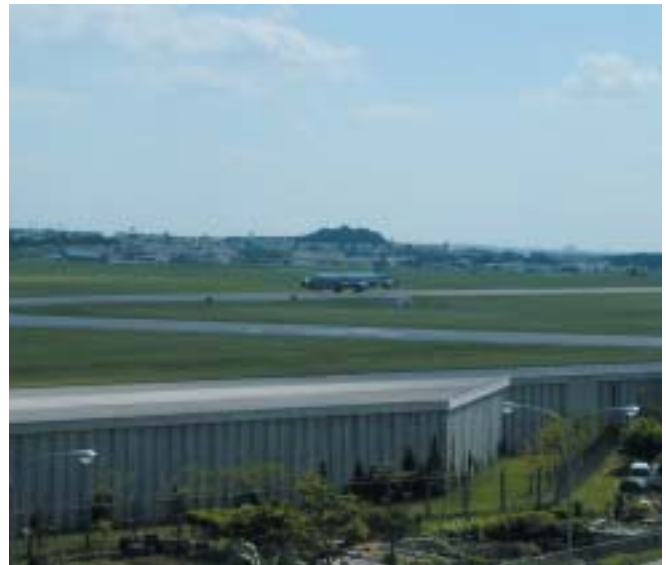
Sound insulation walls installed at the north side of Kadena Air Base as one of the Noise Reduction Initiatives agreed upon in the SACO final report. (at the front of the photograph)
