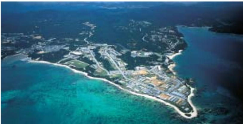
Camp Schwab (the coastal district within the Camp's Water Area at Henoko in Nago City) where work is proceeding for the relocation and return of Futenma Air Station.
